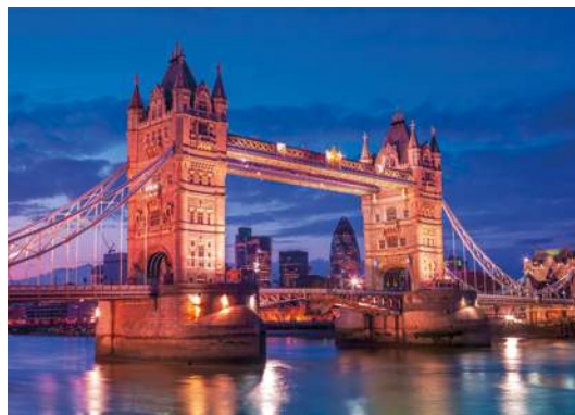
Cod. 39674.0 Tower Bridge
